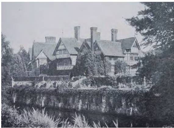
Picture 1.11 Grim's Dyke Hotel 1891
