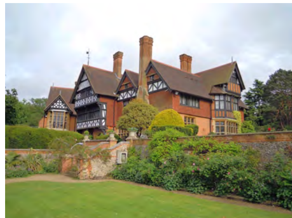
Picture 1.12 Grim's Dyke Hotel 2013
