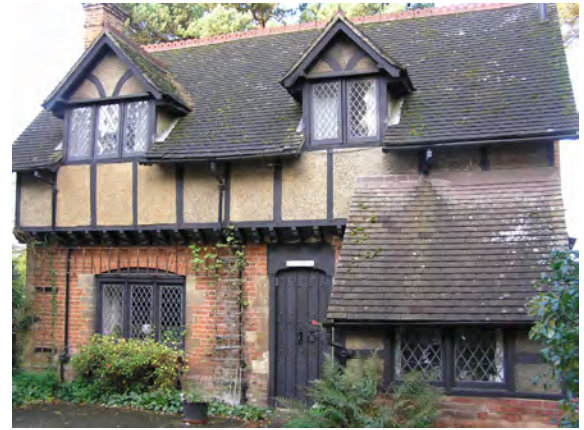
Picture 1.39 North Lodge LBH LA.100019206.2013
